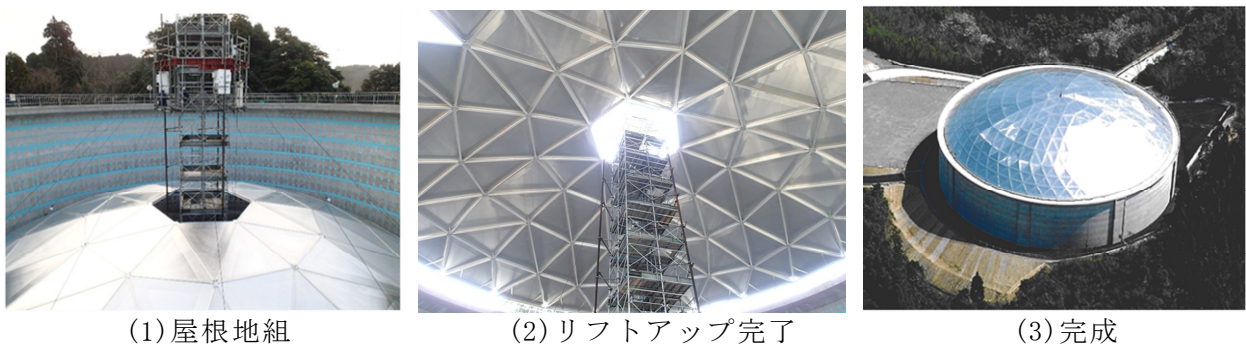
Photo.1 架設、完成状況 Construction, completion status
